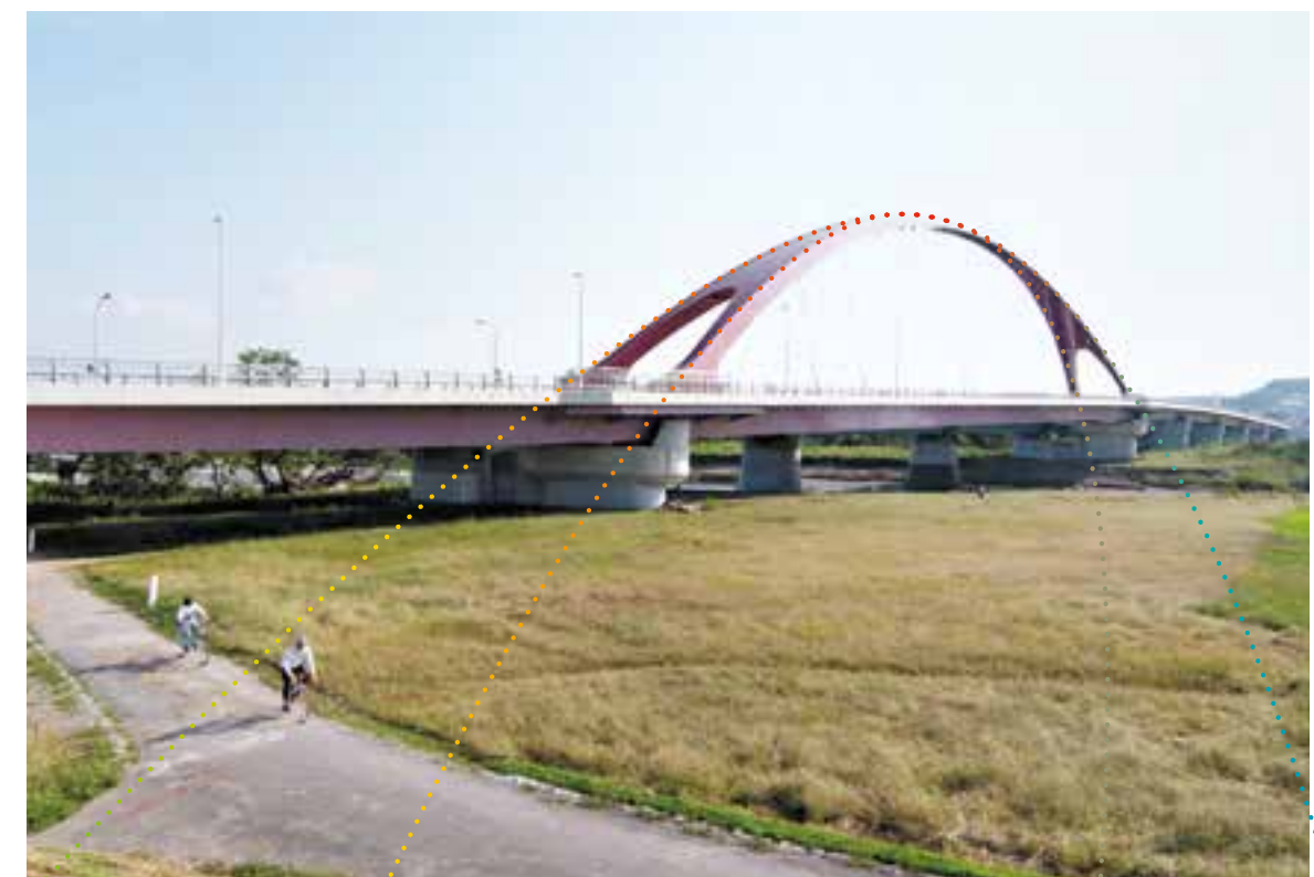
Tama Ōhashi Bridge
